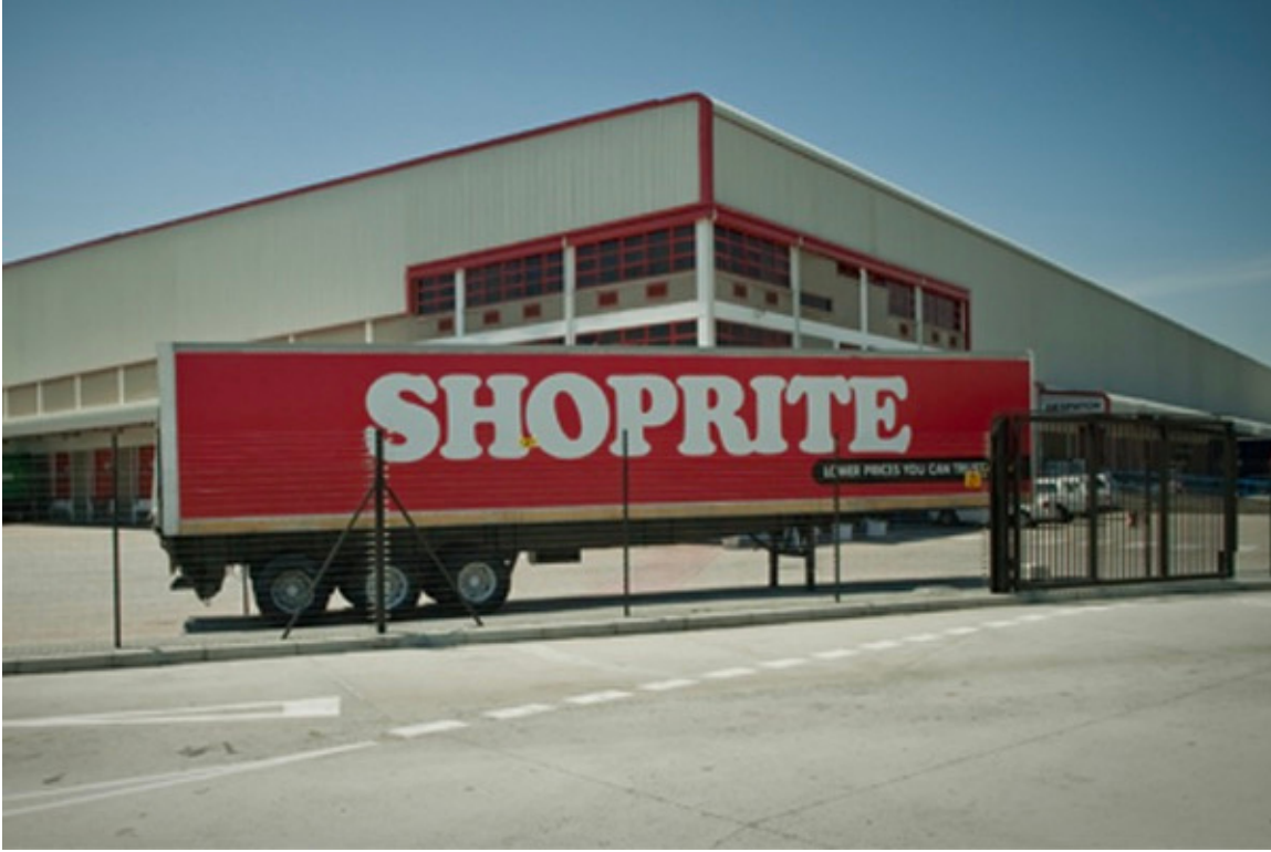
Shoprite distribution Centre Bloemfontein Air Purification for fresh food distribution.
